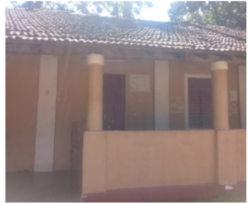
Polling Station Front View
