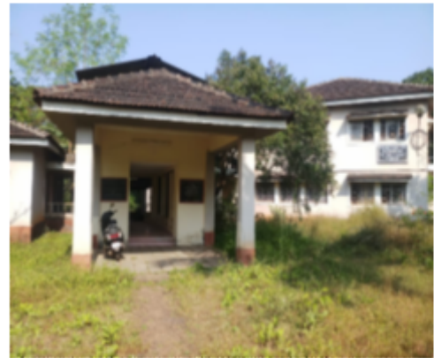
Polling Station Front View
