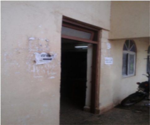
Polling Station Building Front View
