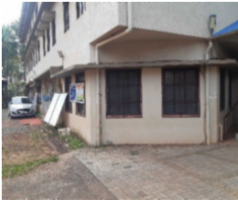
Polling Station Building Front View
