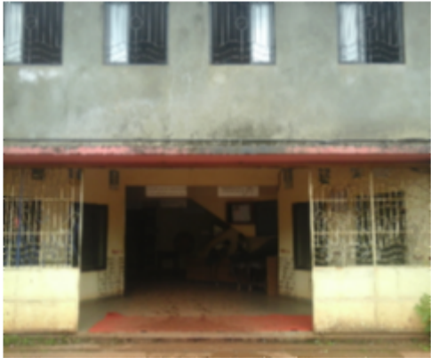
Polling Station Building Front View
