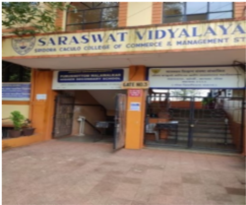
Polling Station Building Front View
