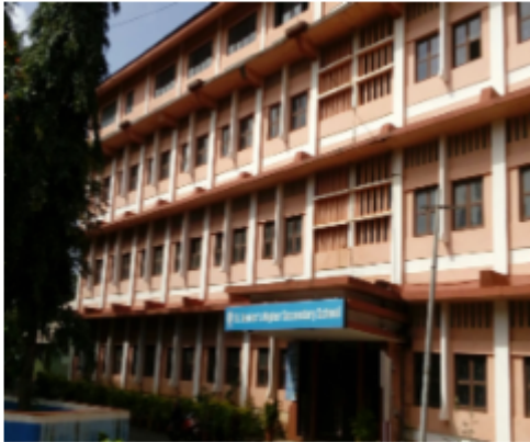
Polling Station Building Front View
