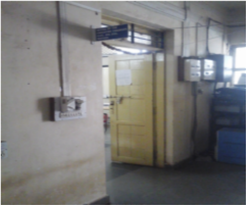
Polling Station Building Front View
