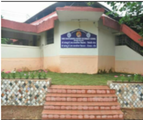
Polling Station Building Front View
