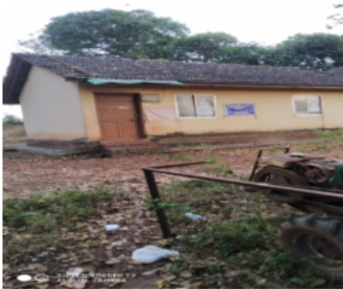
Polling Station Building Front View
