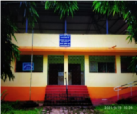
Polling Station Building Front View
